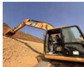
Slope Trimming
