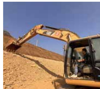
Slope Trimming
