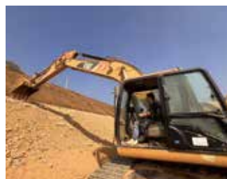
Slope Trimming
