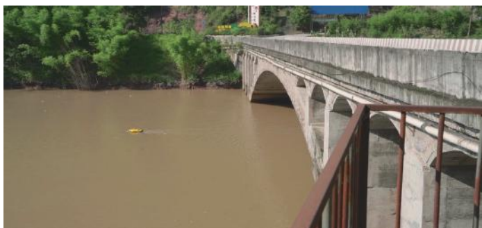
Figure 6. Automated Underwater Survey in Progress
